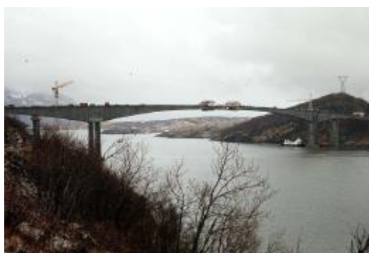
Figure 4.24 Sundøy Bridge in an example of best practice for the free cantilever girder bridges in concrete. Sundøy Bridge is a copy of Raftsundet Bridge that was completed in 1998.
