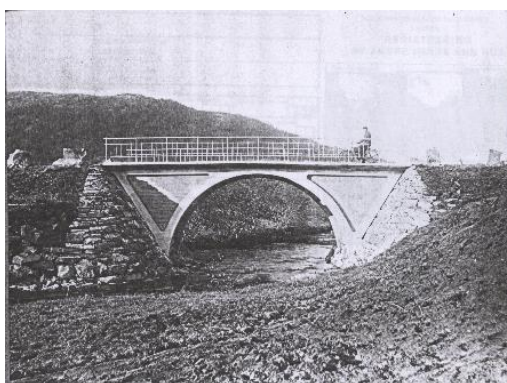
Figure 4.19 The picture above is Leir Bridge in Grong, Northern Trøndelag.
