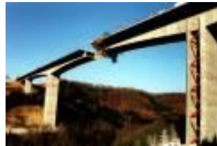
Figure 4.21 free cantilever construction techniques.
